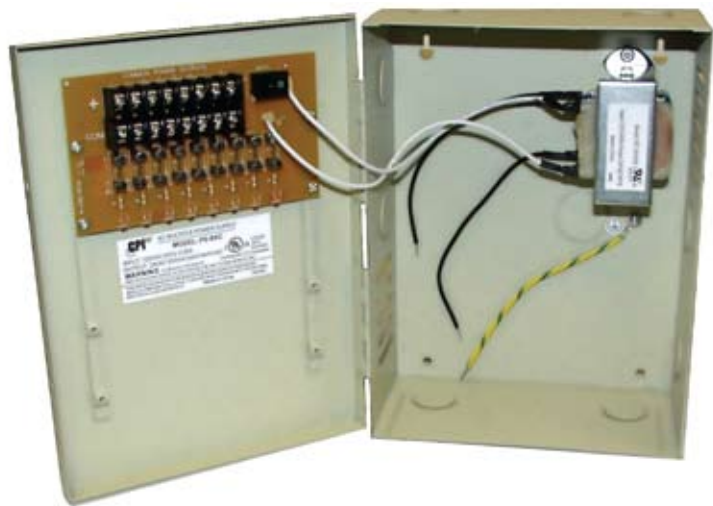
Fig.14 Multi-camera 24VAC power supply
