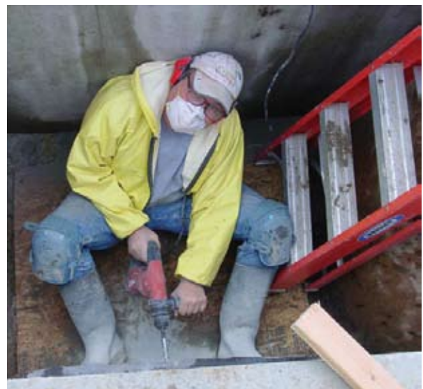
Fig.91 Appropriate protection when drilling concrete
